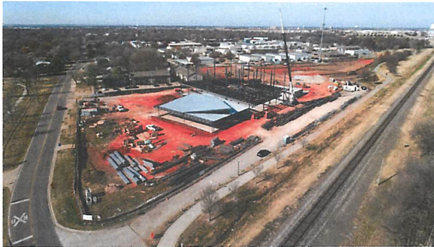
The new Norman Public Library, Central Branch
