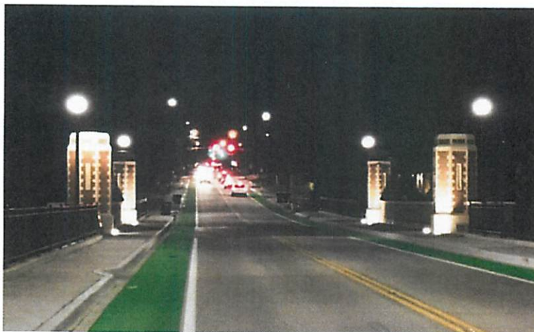
The new West Lindsey Bridge over Imhoff Creek
